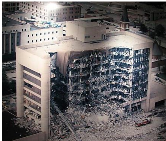
Trümmer des Murrah Federal Buildings 2
